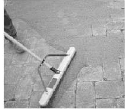
*Figure 5. Joint sand can be pre-mixed and delivered to the site (typically in bags), or mixed with stabilizer at the site, then swept into the joints, compacted for consolidation in them to create interlock, and wetted to activate the stabilizer.*
